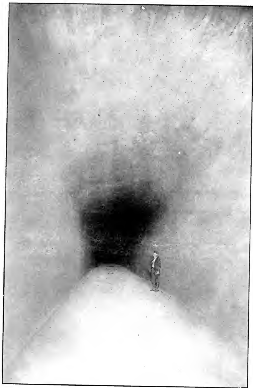
INTERIOR OF TUNNEL NO. 1, TRUCKEE-CARSON PROJECT
